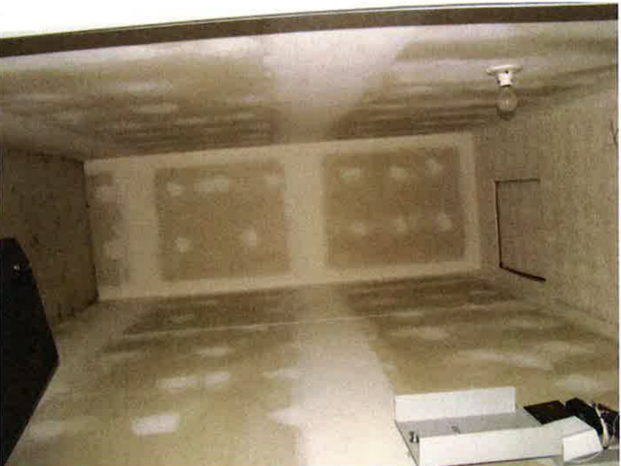
Large closet (Future stairwell to 1 st floor living area)
